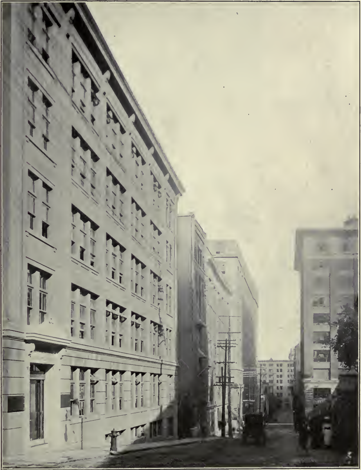
Alexandria Street, looking South. A few years ago this street was occupied by the meanest tenements; to-day it contains some of the finest buildings in the city, and presents a marvel of increased values in real estate.
